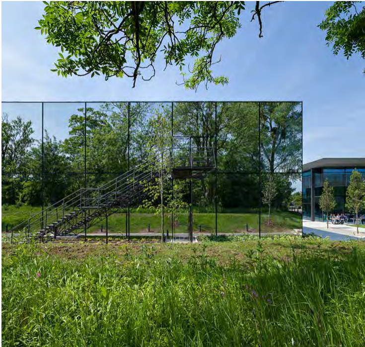
The Dyson Campus in Malmesbury includes the Dyson D9 Research Building complete with its own café. Employees and students certainly can't complain about a lack of greenery.
